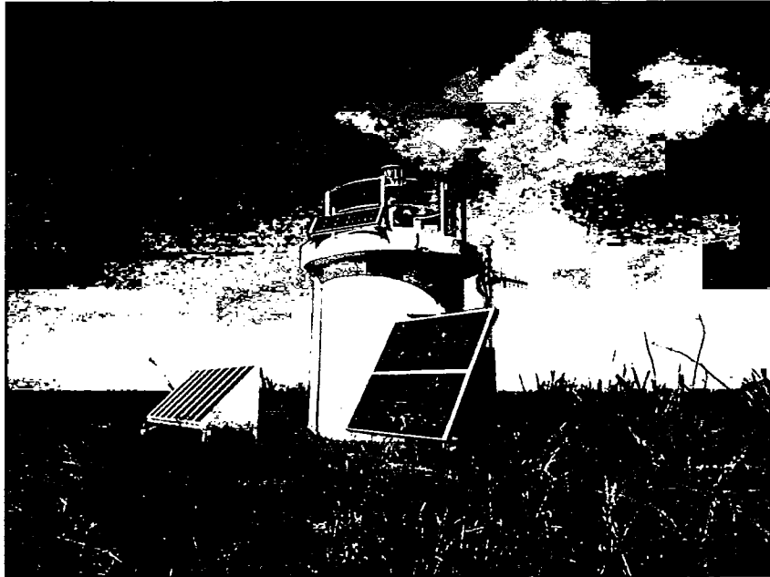
North Cape Tower, Solar Panels and Tsunami Equipment
