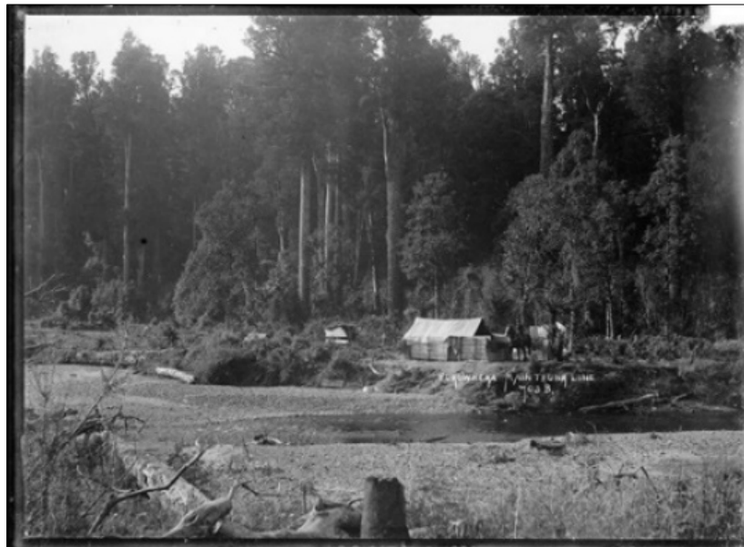
Figure 21: Pukuwheka, on the North Island Main Trunk Railway line (Price, William Archer, 1866-1948 :Collection of post card negatives. Ref: 1/2-000423-G. Permission courtesy of Alexander Turnbull Library, Wellington, New Zealand. /records/23115070)
